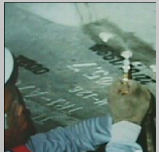
Epoxy Resin Injection
