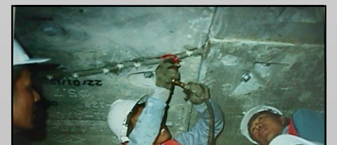
Injection to cracked tunnel segment
