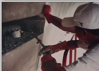
Epoxy Resin Injection
